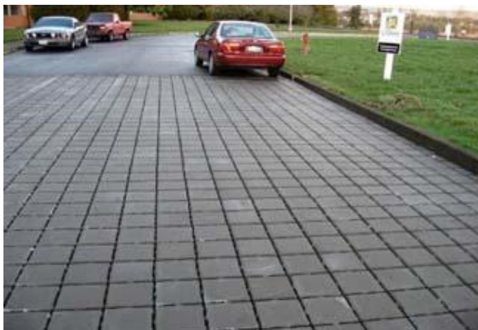
Permeable pavement reduces runoff. Source: epa.gov/green-infrastructure
