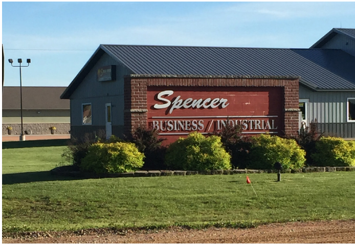
The Spencer Business and Industrial Park Source: Village of Spencer
