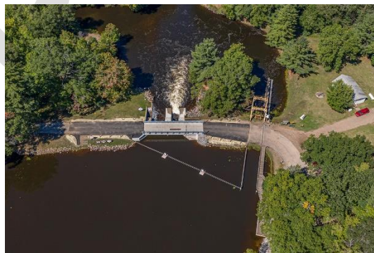
Rollaways Reservoir Dam & Boat Hoist (WVIC)
