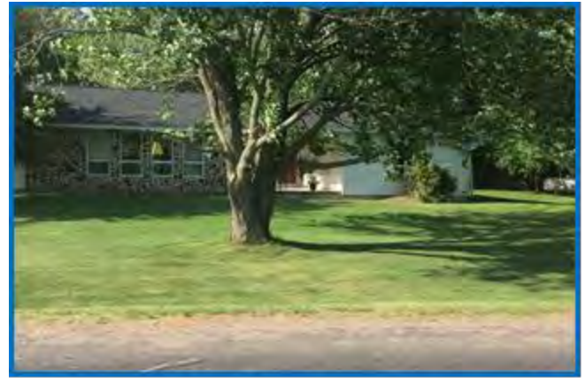
Rural Single-family Home in Maine
