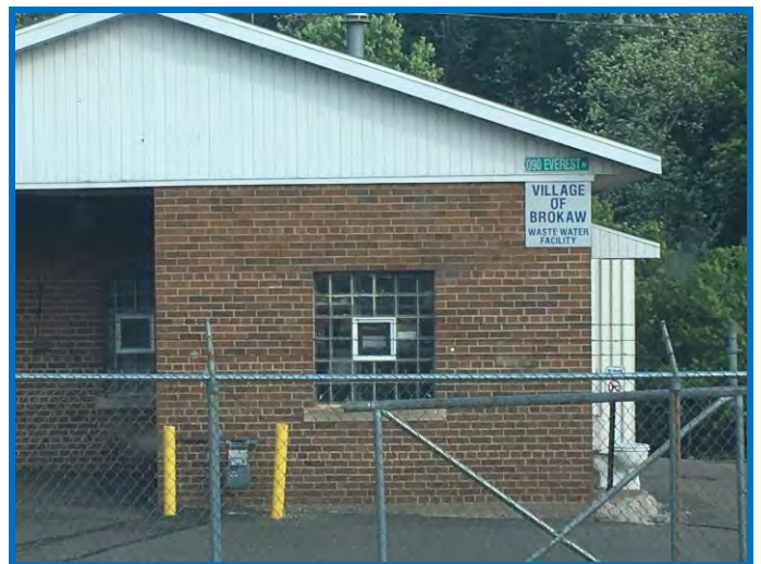
Brokaw's Waste Water Facility
