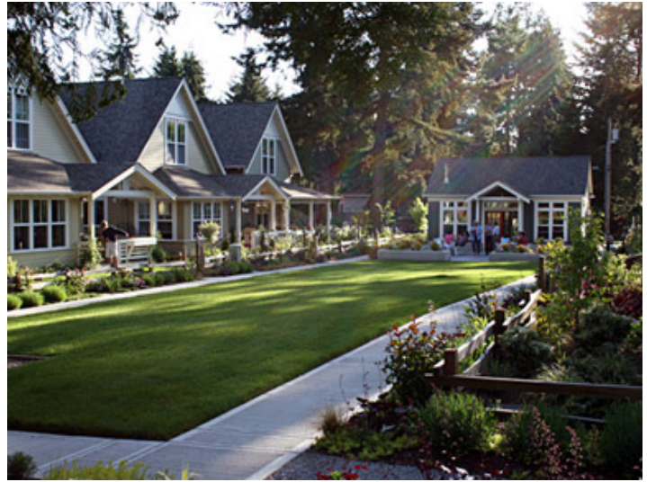
A bungalow court is a high density housing option that can be affordable, low maintenance, and attractive. Image Source: The Cottage Company
