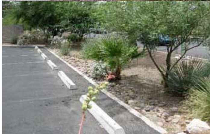
Green infrastructure such as bioswales and rain gardens can be incorporated into streets and parking lots. Source: epa.gov/green-infrastructure
