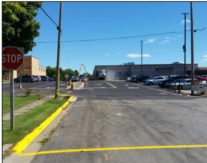
Local roads and parking
