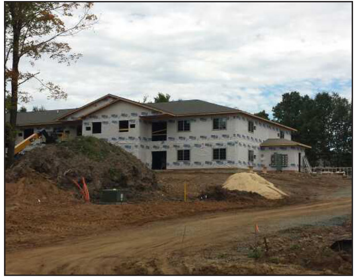
New Multifamily Residential Construction
