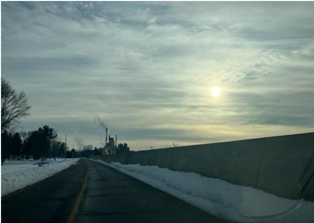
Diking along the Wisconsin River at North Biron Drive
