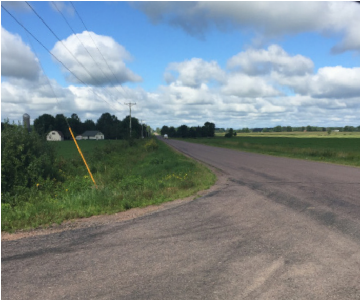
A road paved with blacktop
