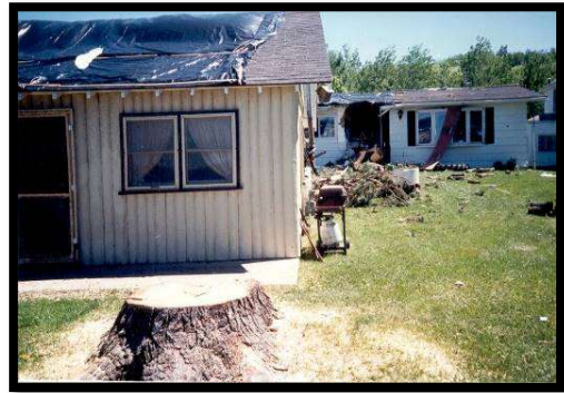
Forest County Tornado Damage, 1994
