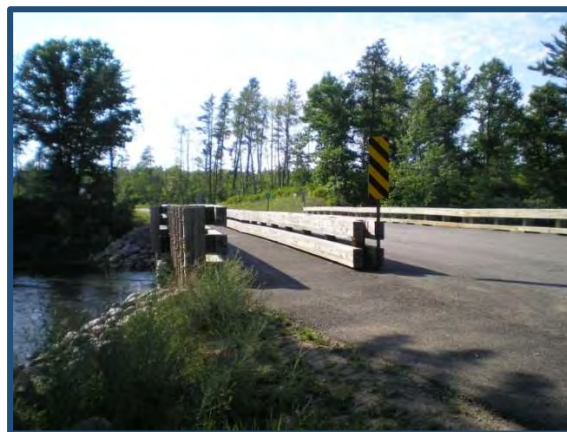
Black Lake Road Bridge
