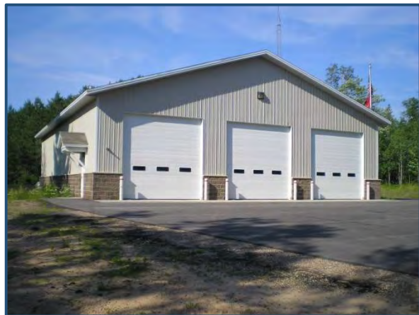
Auxiliary Fire Hall, Twp. 38
