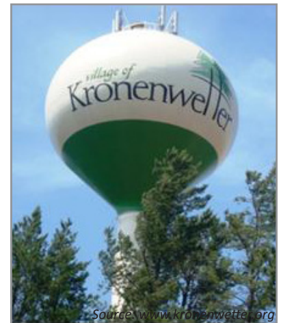
Water towers are an element of a public water utility's infrastructure.
