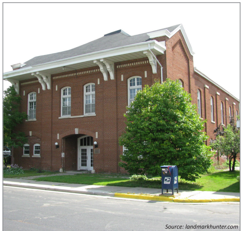
The Edgar Village Hall is on the National Register of Historic Places
