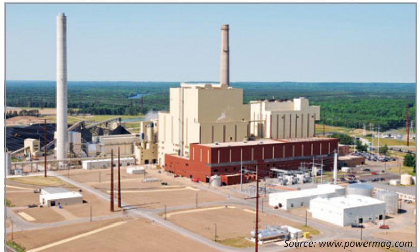
The Weston 4 power plant.
