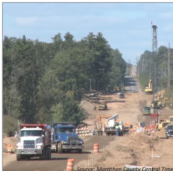
Road construction and repair.
