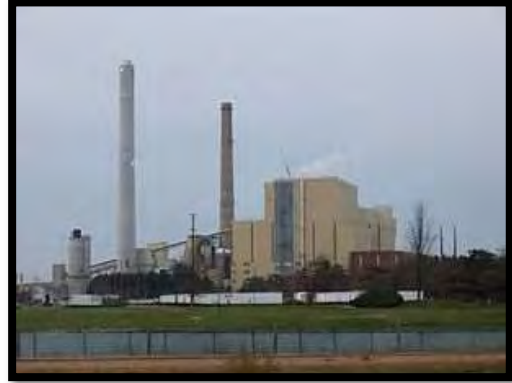
WPS Weston Power Plant
