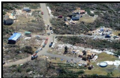
2011 Tornado Damage, Merrill
