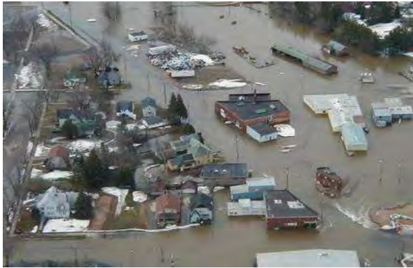
Flooding in Antigo, 2004
