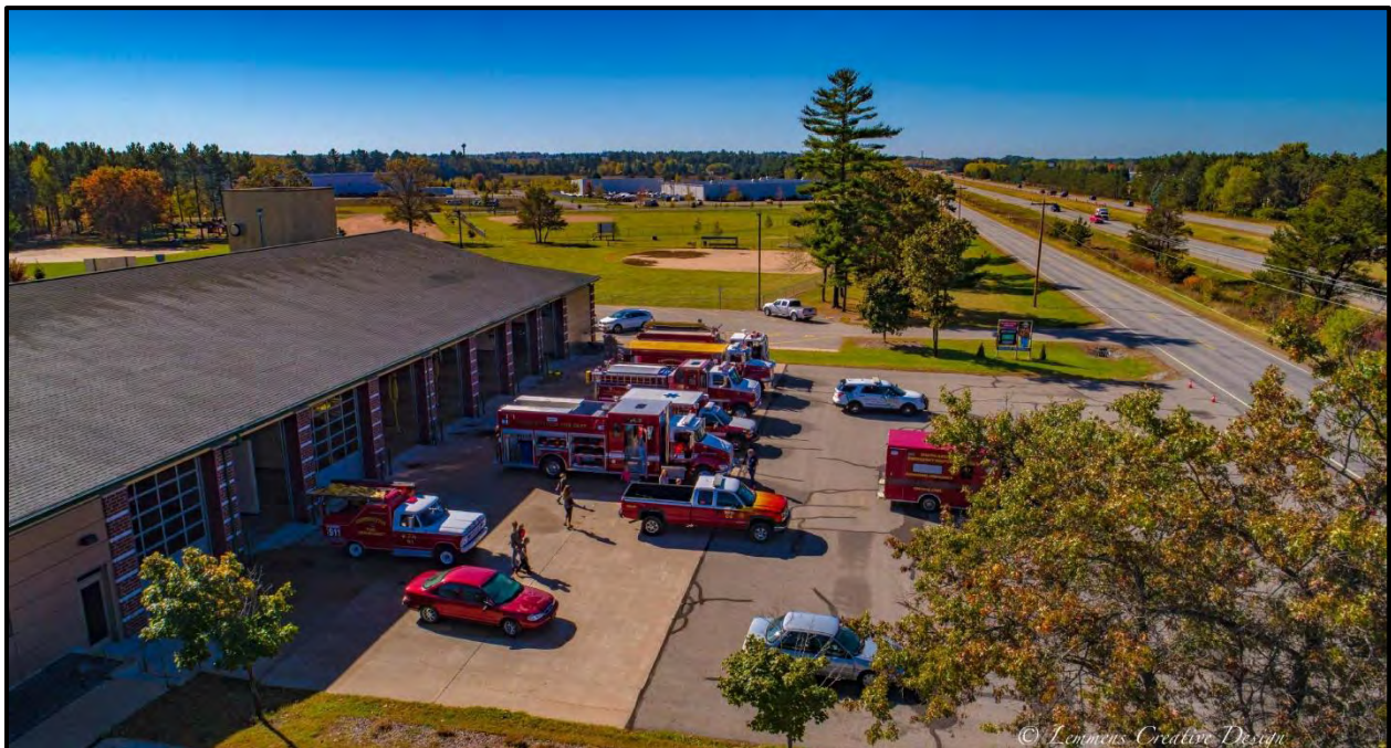
An aerial view of the Kronenwetter Fire Station. (Photo by Lemmens Creative Designs)
