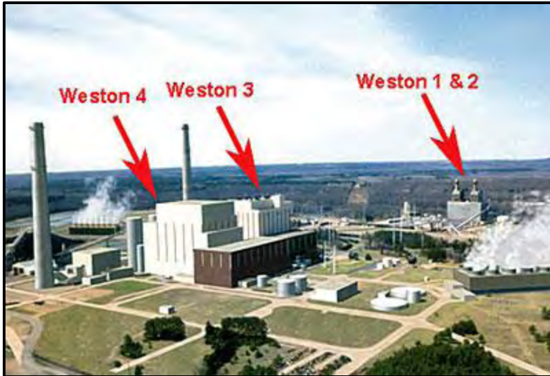
The Weston Power Plant has four operational electric-generating units. Image Source: WXPR Radio
