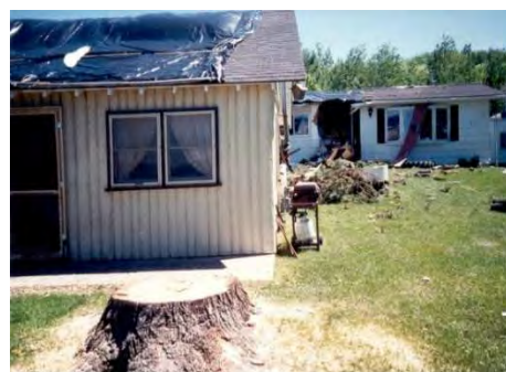
Tornado Damage, Forest County
