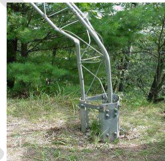
Wind Damage - Com. Tower
