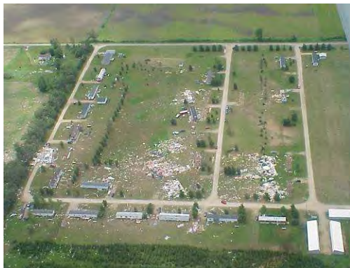
Foster Trailer Park Tornado Damage
