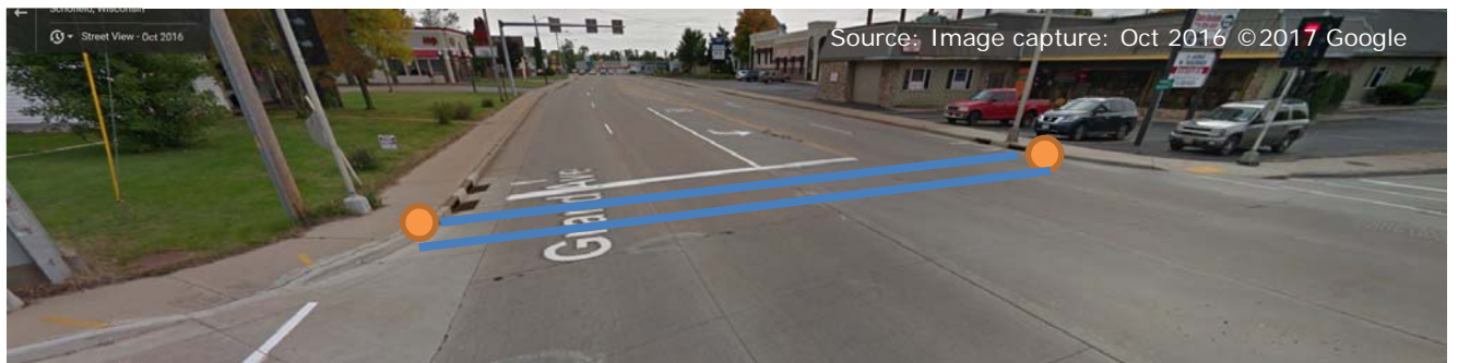
Business 51 and Radtke St, looking south.
