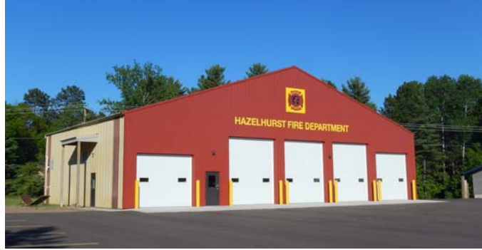
Town Fire Barn
