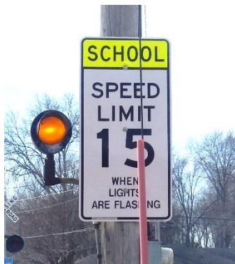
Existing single yellow beacon and School Speed Zone sign assembly
