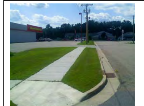
Figure 5 Sidewalk stops at electric poles.
