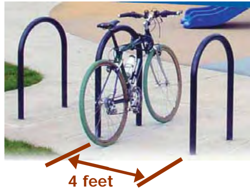
3 inverted U's mounted into the concrete. This rack assembly also parks 6 bikes.
