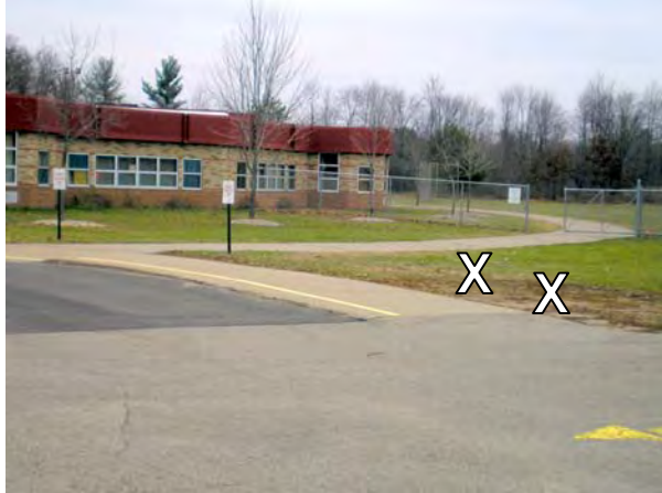
Picture A Install bike racks (Fig 10 or 15) and paver blocks adjacent to the sidewalk in the "X" area.
