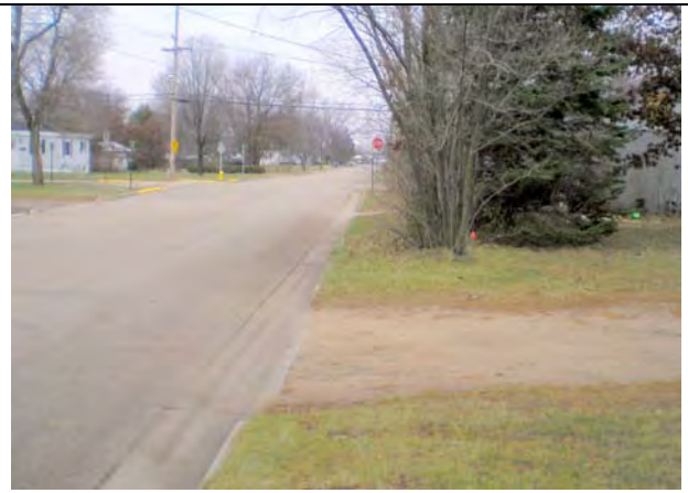
No sidewalk to the east, at the school driveway on Clyde Avenue.
