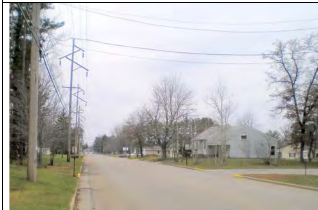
Wide residential streets without barriers promotes traveling faster than the 20 mph school zone speed limit.
