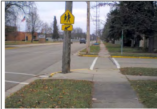
Sidewalks have curb ramps near school. No stop lines painted before crosswalks. Crossing signs are current and properly located.
