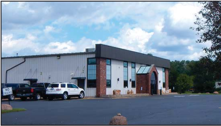
A facility in the Industrial Park.
