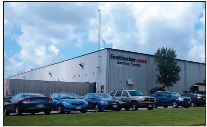
A facility in the Industrial Park.
