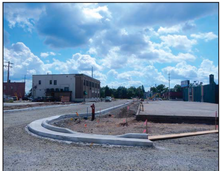
Reconstruction of 2nd Ave.
