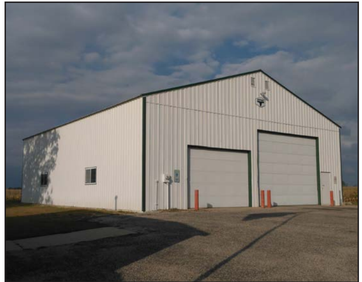
Town of Colburn Garage.
