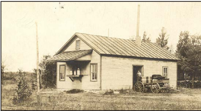
Oakridge Skimming Station
