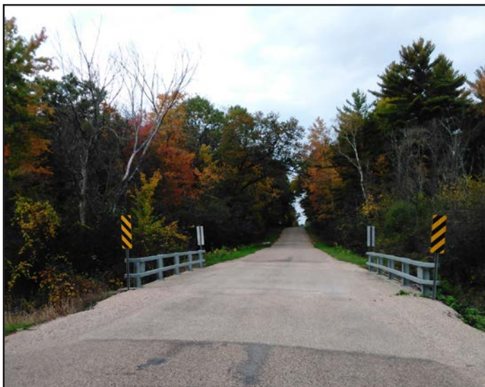
A bridge on 6th Ave.
