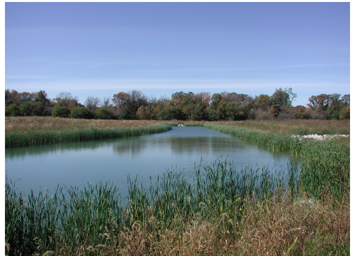
Constructed Wetlands Source: Wisconsin DNR
