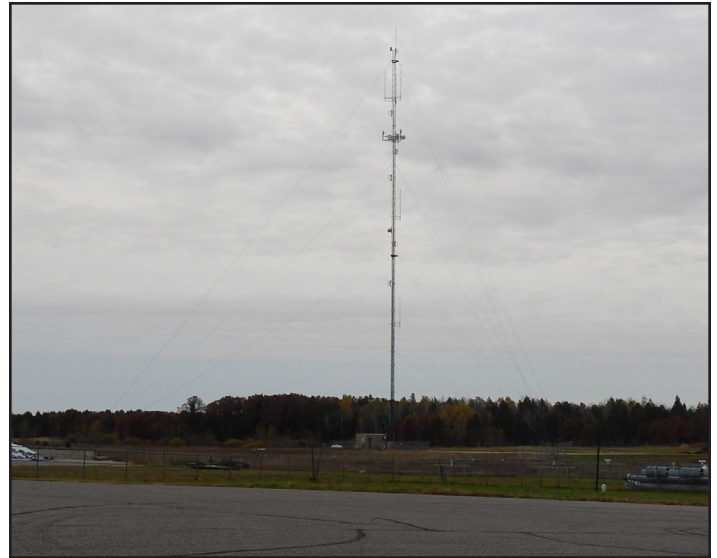
A communication tower.
