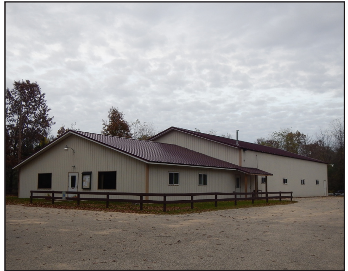
Adams Town Hall Building.
