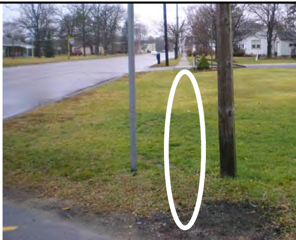
Missing a segment of sidewalk to access school.
