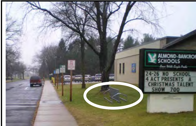
Bike rack is in front of the school. This style of rack was never designed to provide 2 points of contact with a bike for locking and support.
