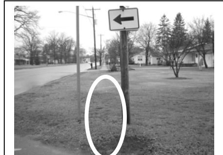
Figure 3 The sidewalk stops, and is missing in an area leading to Bancroft school.
