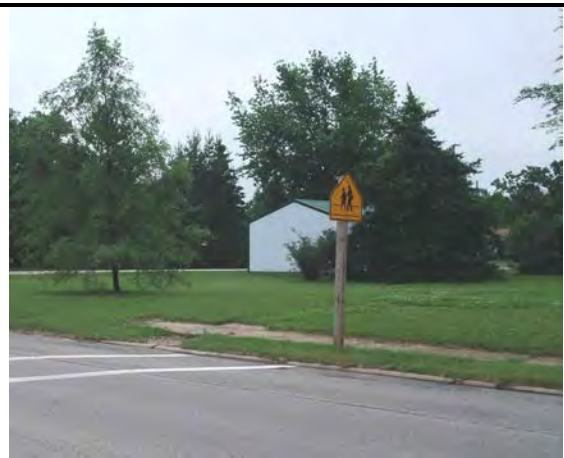
Curb is not handicapped accessible. Crosswalk sign was replaced after picture was taken.
