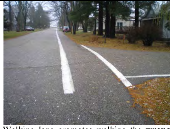
Walking lane promotes walking the wrong way along side of street, because a second walk lane does not exist on the other side.
