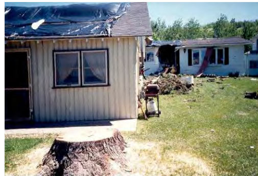
Tornado Damage, Forest County
