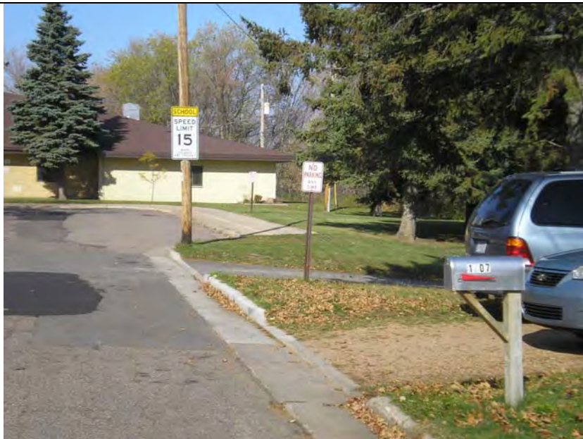
Sidewalk ends. Pedestrian traffic from the south needs to cross Fulton St twice to enter front door.
