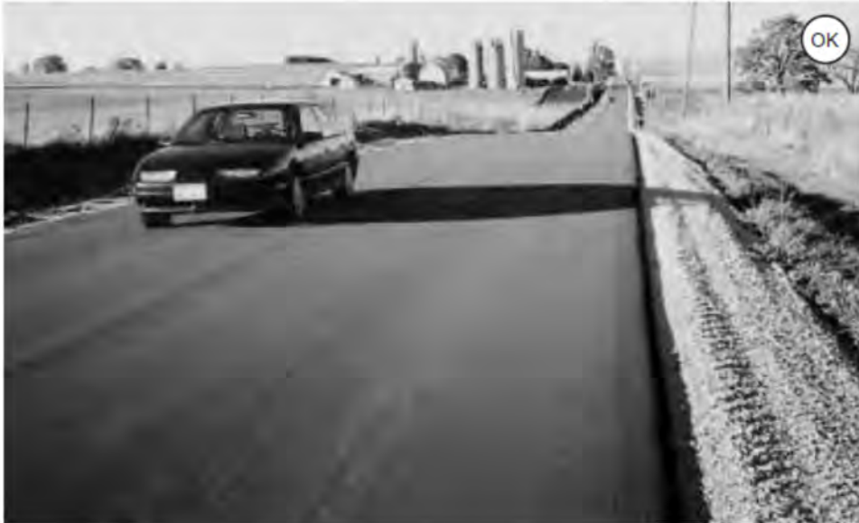
Figure 2-9: Many low-volume country roads need few improvements in order to serve bicyclists well.
