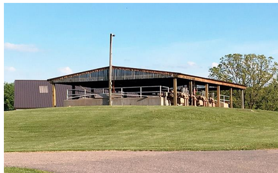
Village of Hatley Wastewater Treatment Facility Source: Village of Hatley
