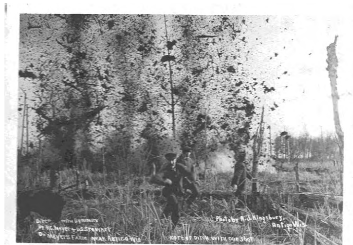
Drainage Ditching via Dynamite in the Early Days
