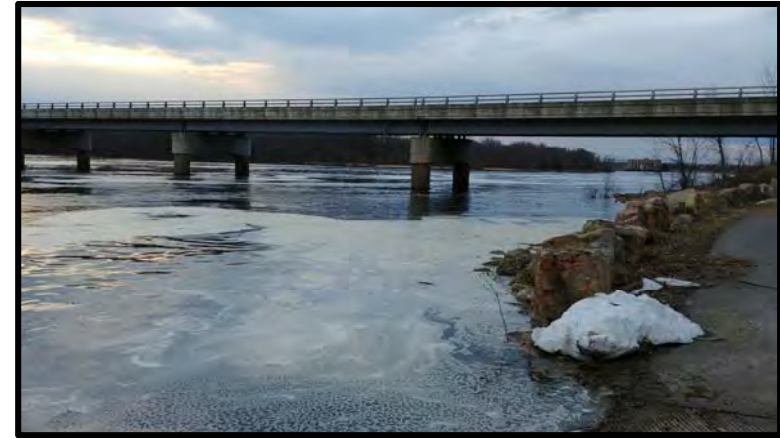
The State Highway 21 Bridge over the Wisconsin River connecting Adams and Juneau Counties. Image source: NCWRPC
