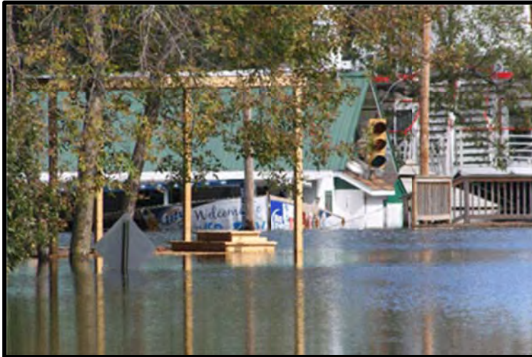
River Bay Campground in the Town of Lyndon experienced flooding with water levels exceeding 9-feet in 2010 Image source: Wisconsin Dells Events
