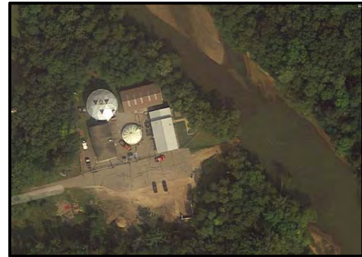
An aerial view of the Necedah Wastewater Treatment Plant.
