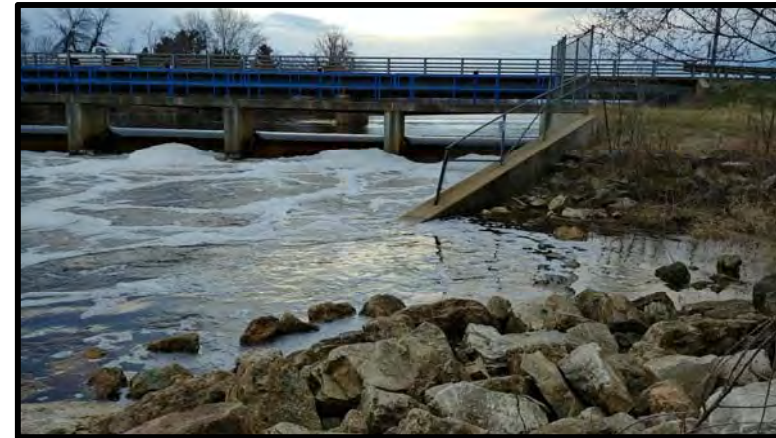
High water at the Necedah Dam in Spring 2018.
