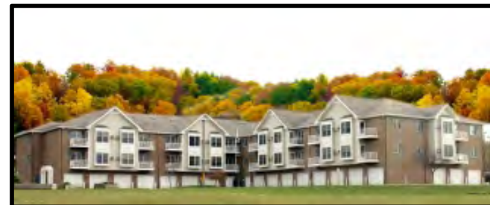
Flooding near nursing homes like Terrace Heights in Mauston can put citizens in harm's way. Image source: Mile Bluff Medical Center
