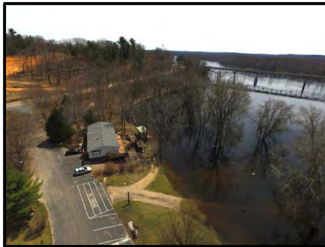
Flooding can disrupt or completely stop business operations, such as for this campground and resort. Image source: Rocky Gilner
