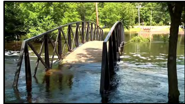
Flooding at Friendship Park in 2017. Image source: FOX6NOW
