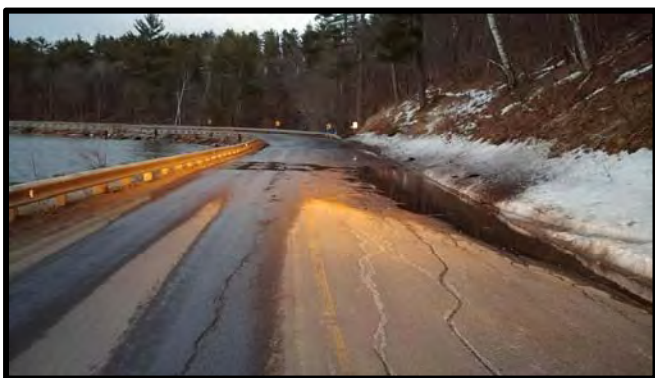
A flooded portion of County Highway Z in Adams County during Spring 2018. Image source: NCWRPC
