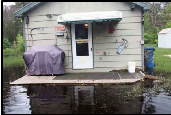
Heavy rains caused this property in Clearfield to flood with standing-water levels approaching 2 feet.
