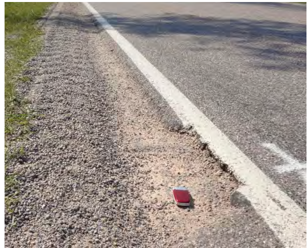
Maintain gravel edge to reduce bicycles tipping as they use the shoulder for safety
