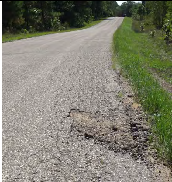
Alligator cracking road Soon potholes will develop (as seen)
