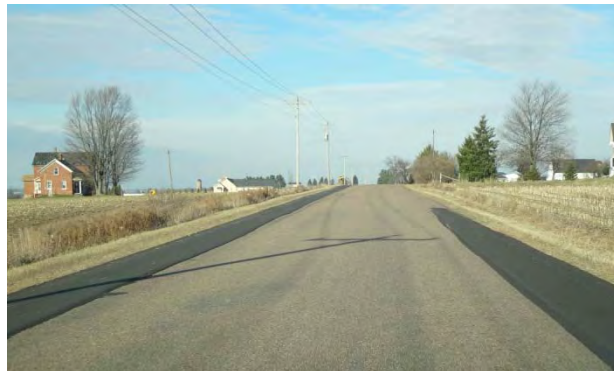
Edge patching may cost effectively extend the road life to accommodate bicycles and motor vehicles.
