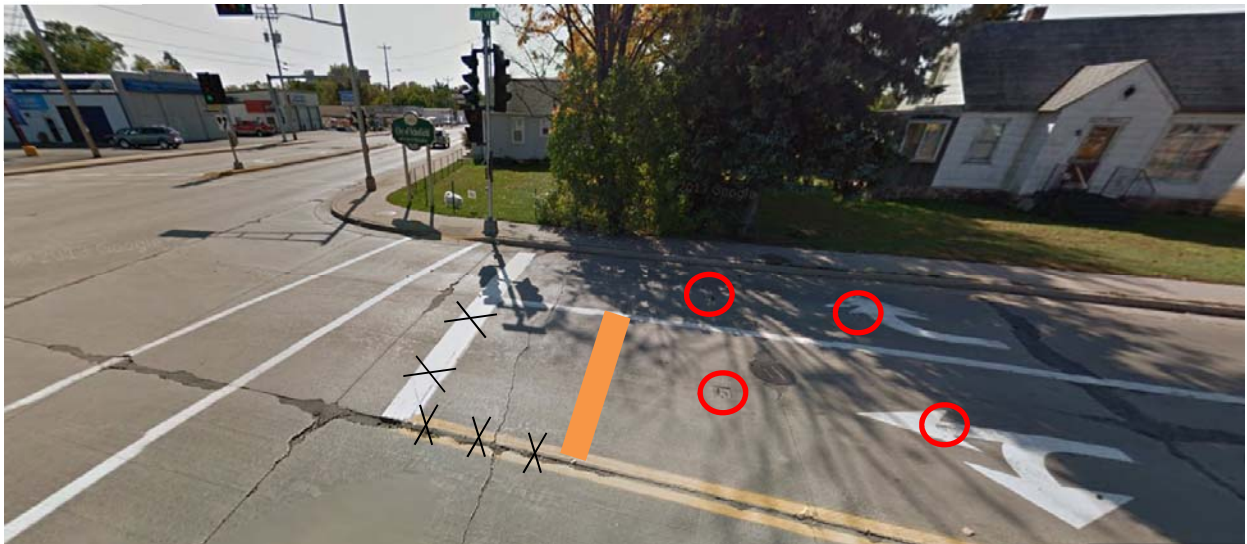
Eastbound Lake View Drive at Business 51
