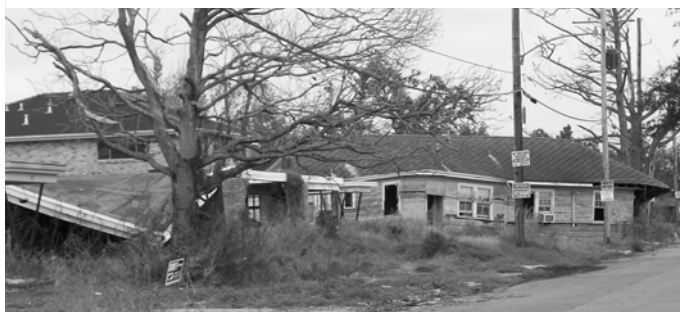
Near the 17th Street Canal
