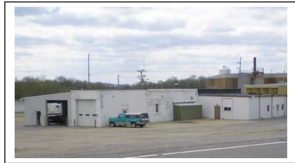
Town Hall & Garage
