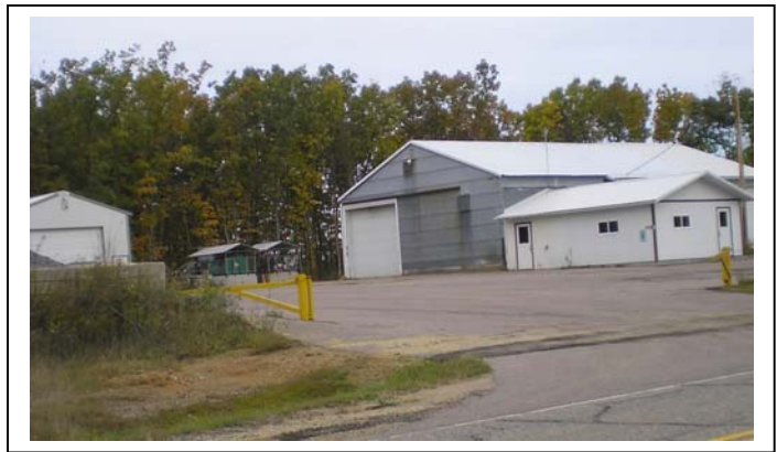
The Town of Summit maintains shop facilities along STH 58 where it stores road equipment and supplies.
