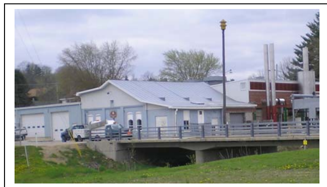
Municipal Garage also contains electric generating equipment
