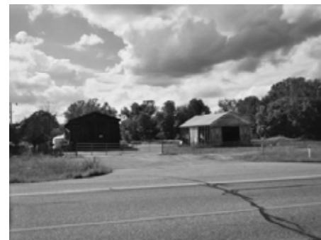
Adams County Highway Department Barns on STH 13
