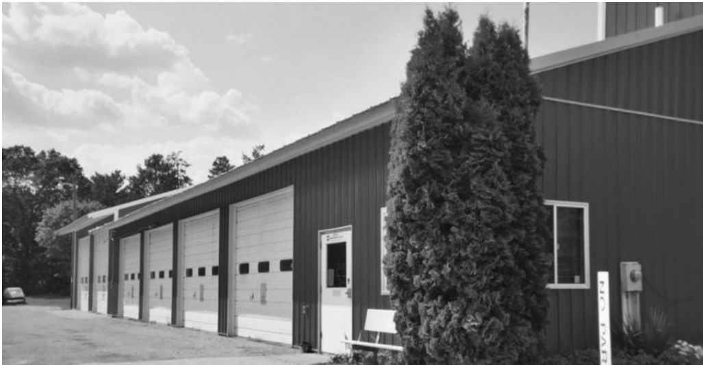
Fire Hall – Town of Quincy
