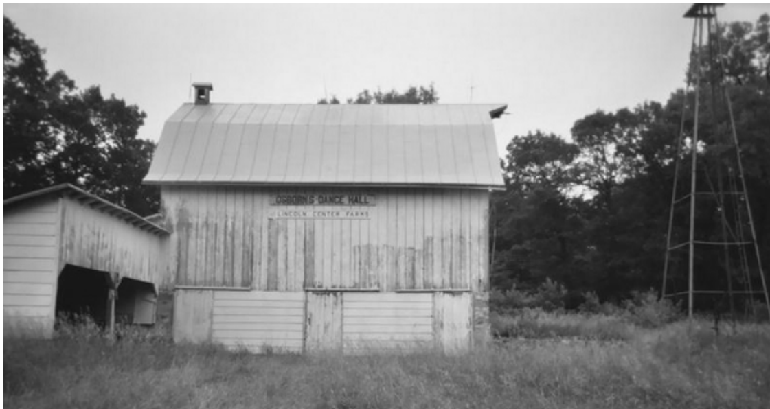
Lincoln Center Farms barn – Town of Lincoln
