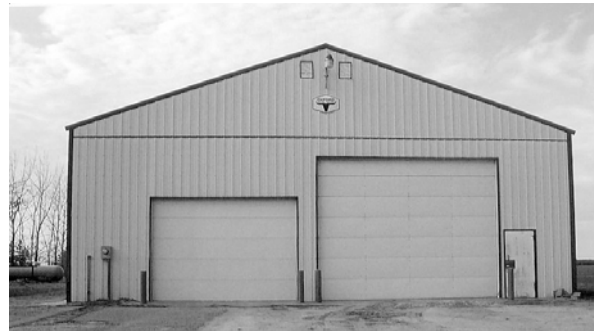
Town garage – Town of Colburn
